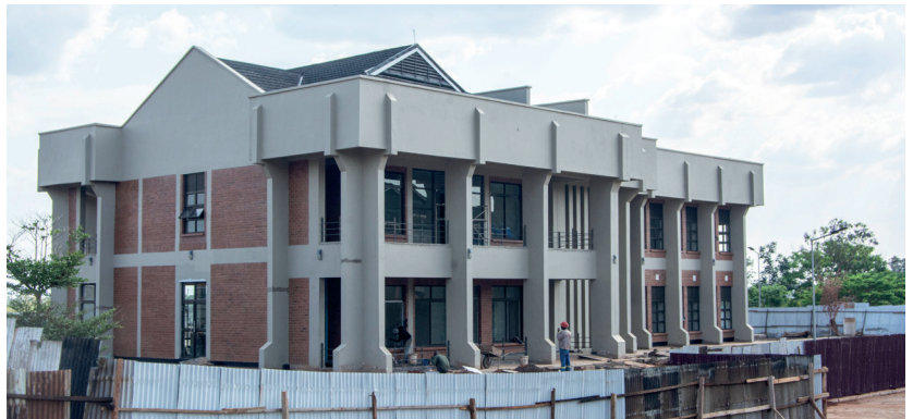
The AquaFish Office Complex under construction
